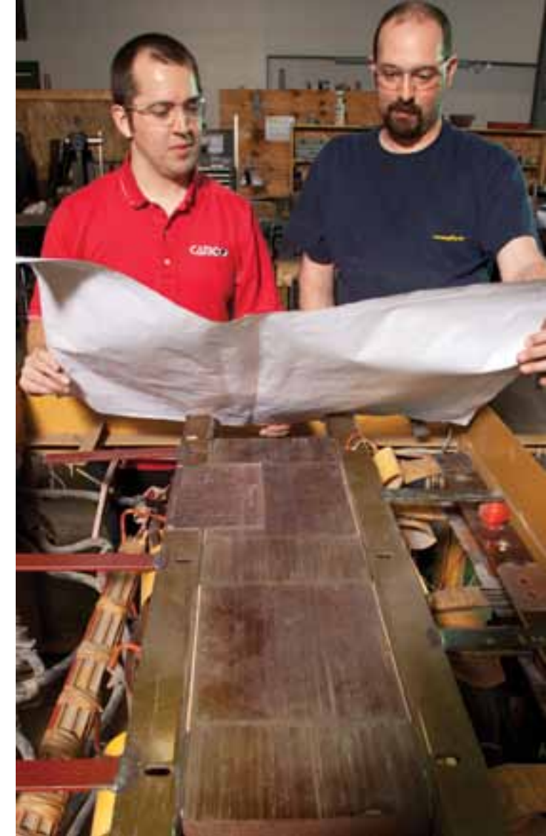
CAMCO Technicians Chris Keilman and Jeff Giffin checking power center wiring to the schematic.
